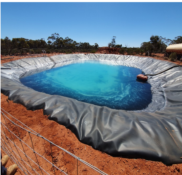
Dust suppression dam on Battery bore field line
