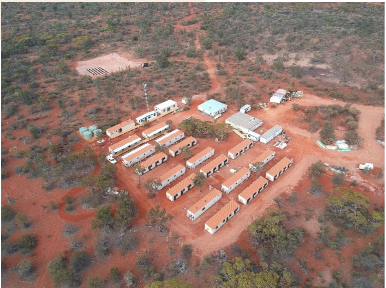
Riverina camp nearing completion at quarter end
