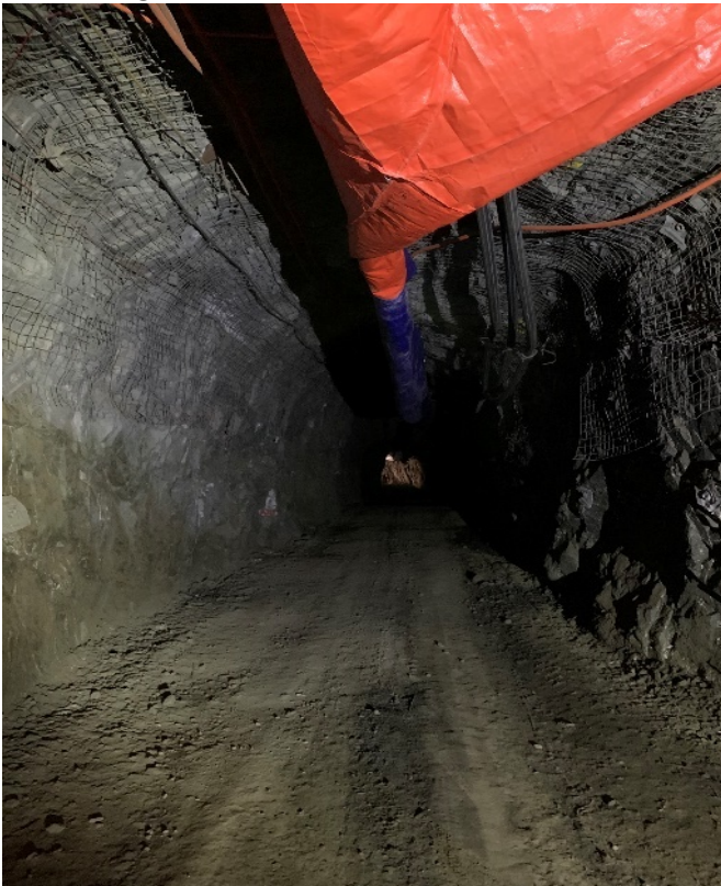
Re-establishing decline ventilation
