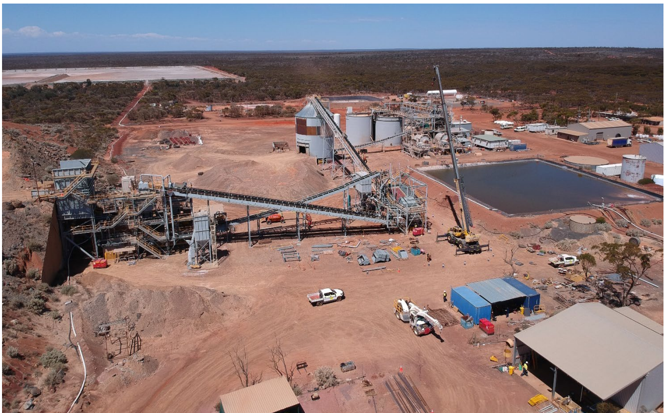
Process plant remedial works in progress during the quarter
