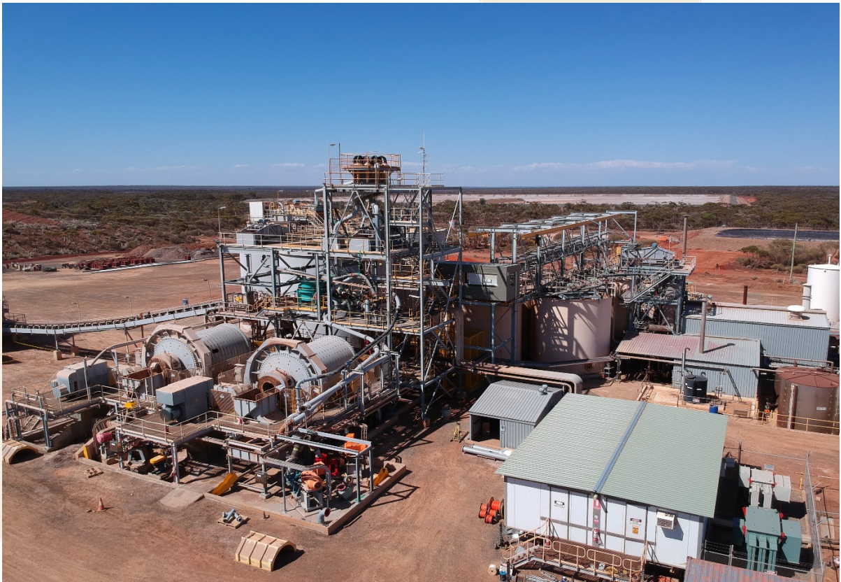
Process plant remedial works in progress
